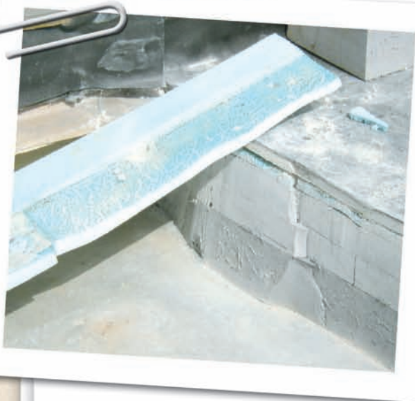
Figure 4: Melted XEPS.
