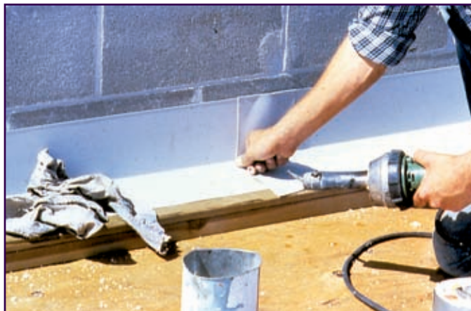
Figure 13: Polymer-coated metal flashings anchor this PVC roof membrane system.
