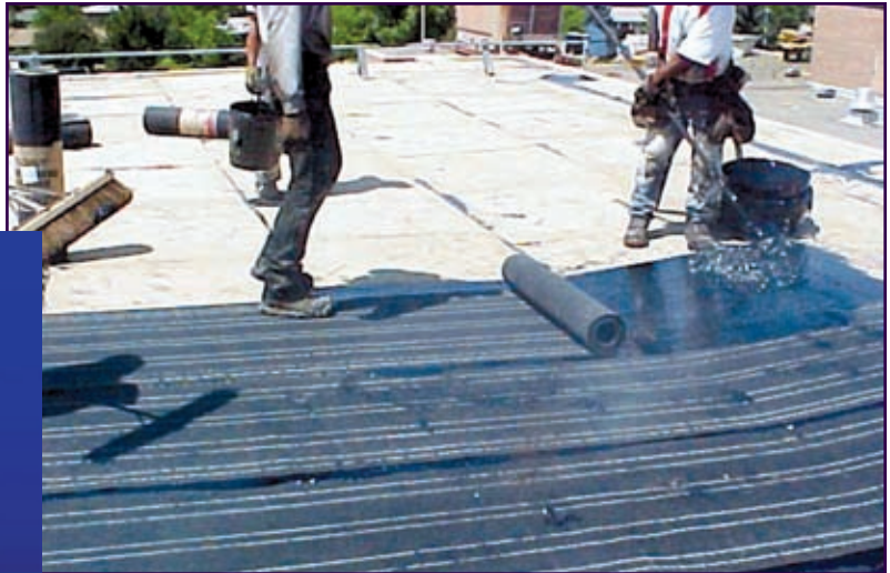
Figure 4: The field-applied bitumen serves both as adhesive and waterproofing agent.
