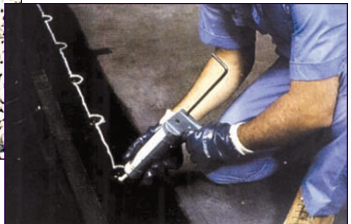
Figure 22: Use of in-seam sealant as extra measure against water penetration.
