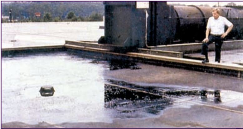
Figure 23: Polyepichlorohydrin rubber was used in this roof bay in order to resist oil contamination.
