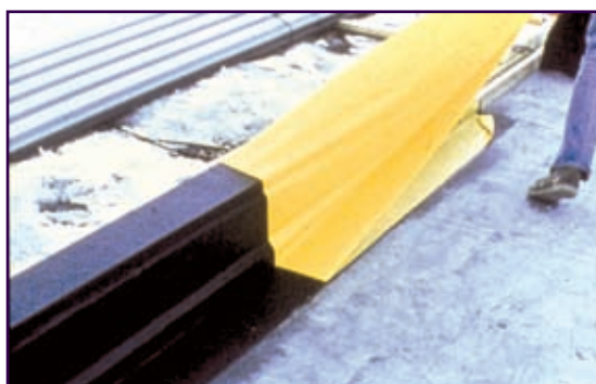
Figure 11: Uncured neoprene sheeting provided the conformability needed for flashings and penetrations.
