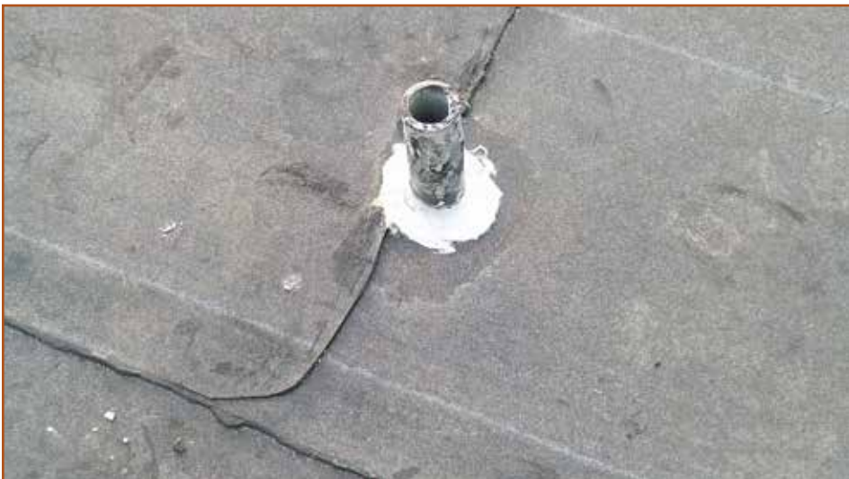
Photo 8 – Sealant applied around penetration on modified bitumen.
