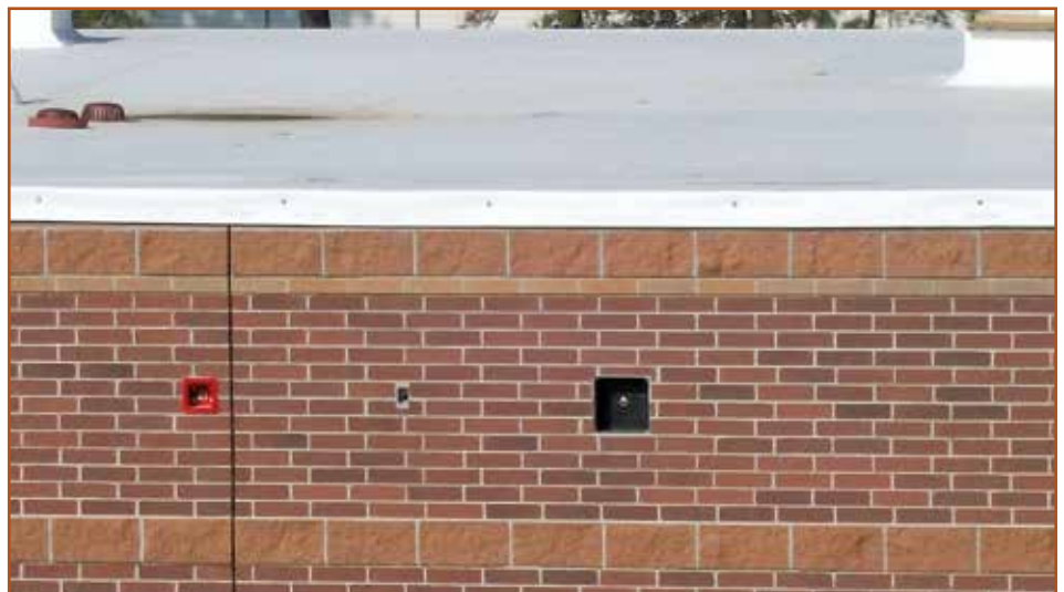
Photo 10 – Trimmed edge of single-ply at perimeter.
