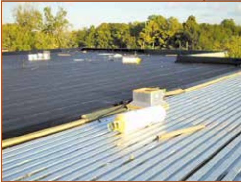
Photo 5 – Tie-in of modified bitumen on metal deck.
