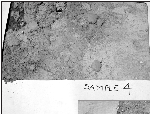
Photo 1 – Moisture-damaged gypsum cover board.
