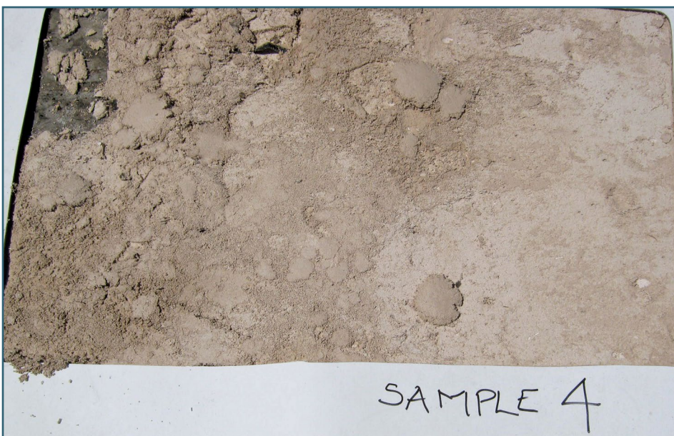
Photo 1 – Moisture-damaged gypsum cover board.
